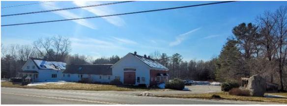
640 Maple Street, Contoocook, NH, An 1880 farmhouse on 5.5 acres near Exit 6, I89 that was converted into eight residential units
