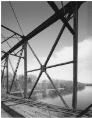
NH-669-21. Detail of truss posts, diagonals, and bracing connections. Looking east.
